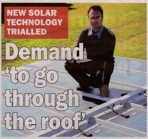
GAME CHANGER: Dr Dragos Petrescu demonstrates the weight-bearing capabilities of the integrated photovoltaic roofing panel he designed.
